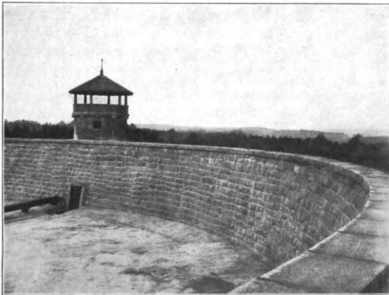
FIG. 2. FINISHED WALL, INLET PIPE, AND OUTLET SCREEN.
