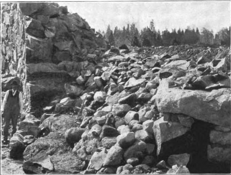
FIG. 2. DRY MASONRY OUTSIDE WALL AND DRAIN.
