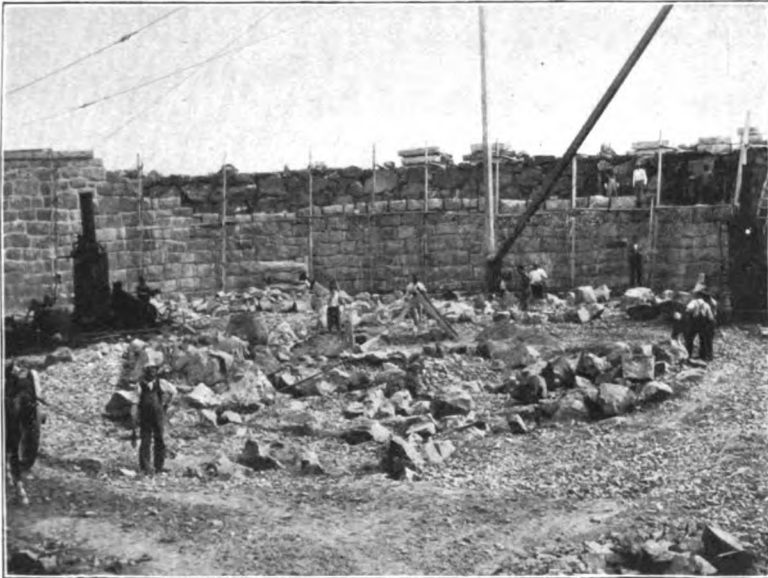
FIG. 1. EXCAVATION OF LEDGE, AND CONSTRUCTION OF OUTER AND INNER WALLS.
