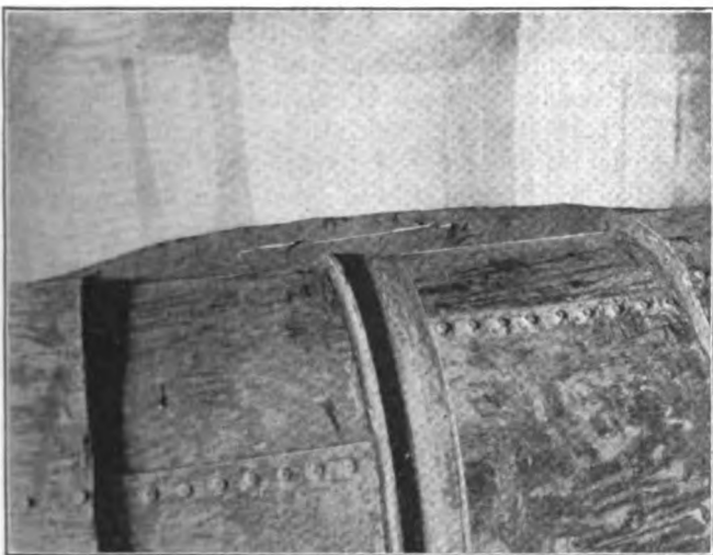
FIG. 7. COMPLETED JOINT IN CEMENT-LINED MAIN WITH CONCRETE COATING REMOVED
