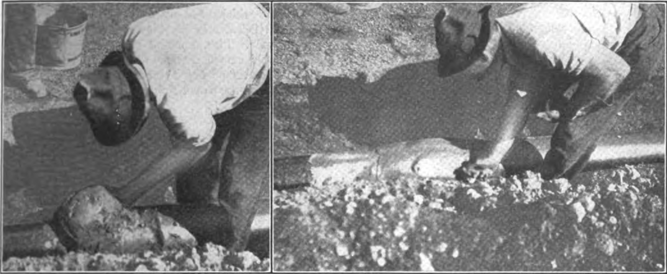
FIGS. 5 AND 6. COVERING THE JOINT WITH NEAT CEMENT MORTAR
