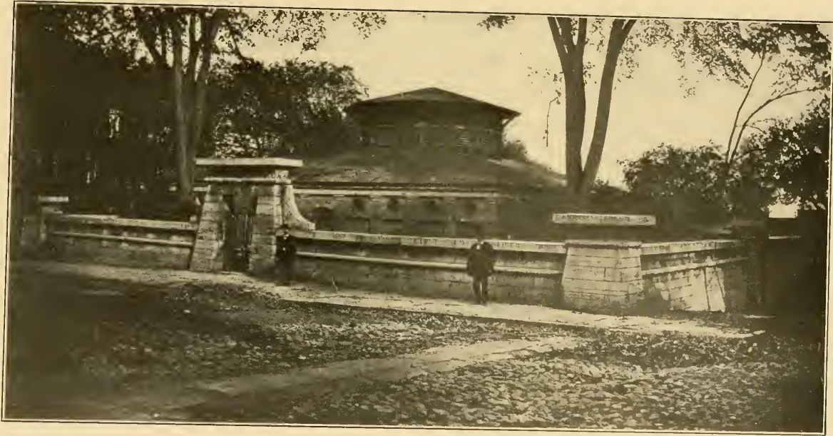
WATERWORKS COMPANY RESERVOIR.
