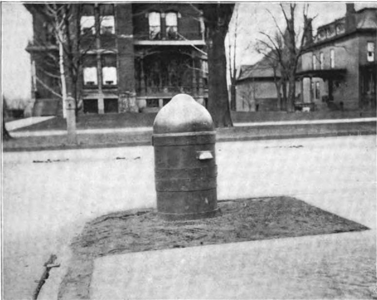
**FIG. 2. — HYDRANT WITH STEEL COVER.**
