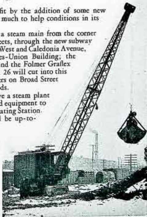
One of the Company's large locomotive cranes breaking ground for Station 9 Steam Plant, Lincoln Park.
