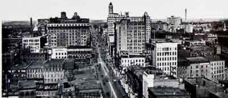
With more than 300 private boiler plants and their smoking chimneys discontinued in favor of the Company's steam service, the effect upon Rochester's skyline is becoming noticeable. Central station steam service is a constructive contribution toward smoke prevention.
