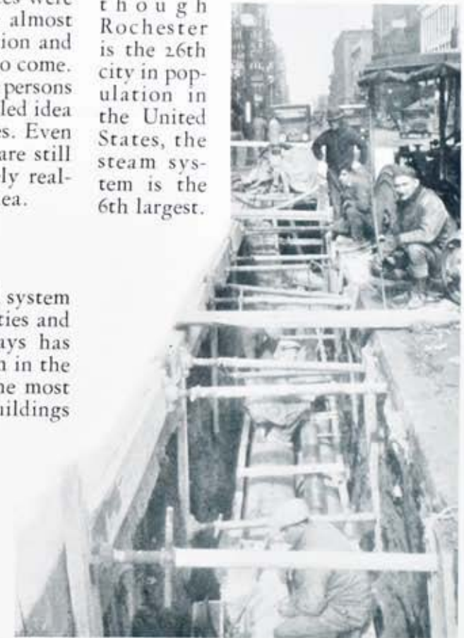
Progress of underground steam construction. Electric welding crew has completed installation which consists of three pipes at this location: a 14-inch low pressure steam main; an 8-inch high pressure steam main and a 6-inch pipe through which the condensed steam is returned to the station. Insulation crew is at work in preparation for the final construction of concrete box forms, back fill and re-paving.
