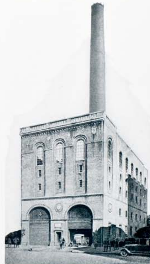
The commercial district heating plant Station 8, Lawn Street at the rear of the R. G. and E. Bldg. This modern powdered coal steam generating plant serves all of the new buildings and many other customers in its district in the downtown section of Rochester.
