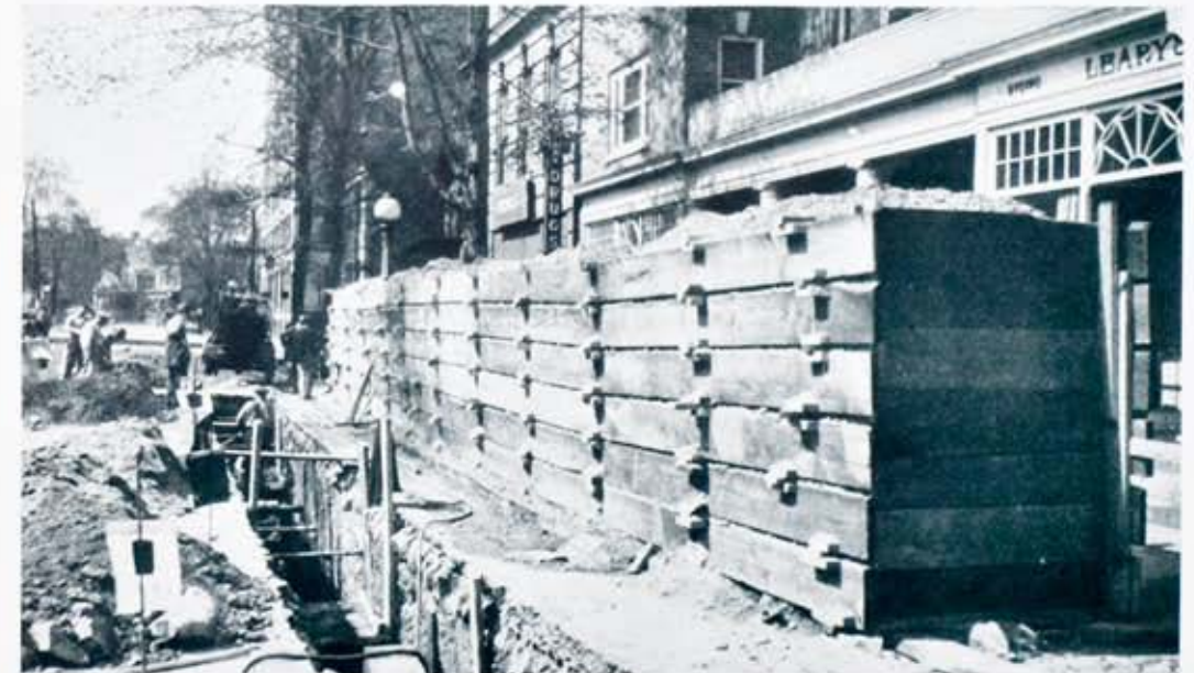
Steam construction in progress in Chestnut Street. This view shows the method used in caring for the dirt removed from the trench, and to avoid interference with pedestrian and vehicular traffic and in the interest of safety. This dirt is used later for back-filling the trench.
