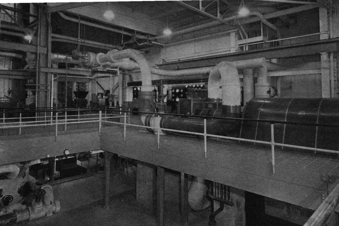
Fig. 1. General appearance of operating room. The 250,000 lb. steam generating unit is at the left; the 6000 kw. turbine at the right and the control board in the central background. Note method of anchoring steam line
