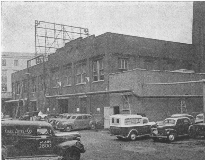
FIG. 6.—Main Emerging from Building at Left Runs Along Outer Wall of Substation Through Expansion Loop Before Entering Desuperheater House.
