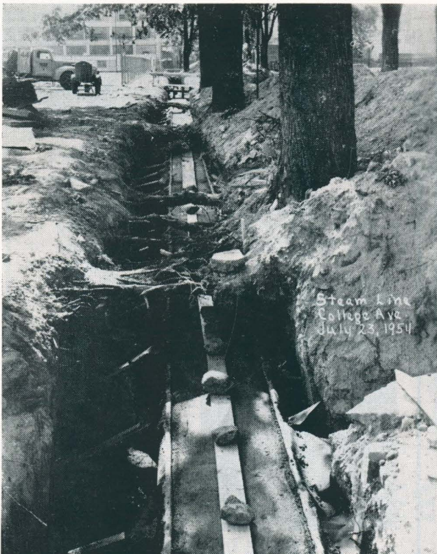
Steam Line—College Ave., July 23, 1954
