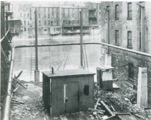
FIG. 2 — Expansion loop in 12-in. high pressure main, in process of construction in 1945, which was reconstructed in new location in 1968, due to urban development program.
