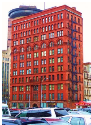
Figure 4. Wilder Building located at 1 E. Main Street, Rochester.
