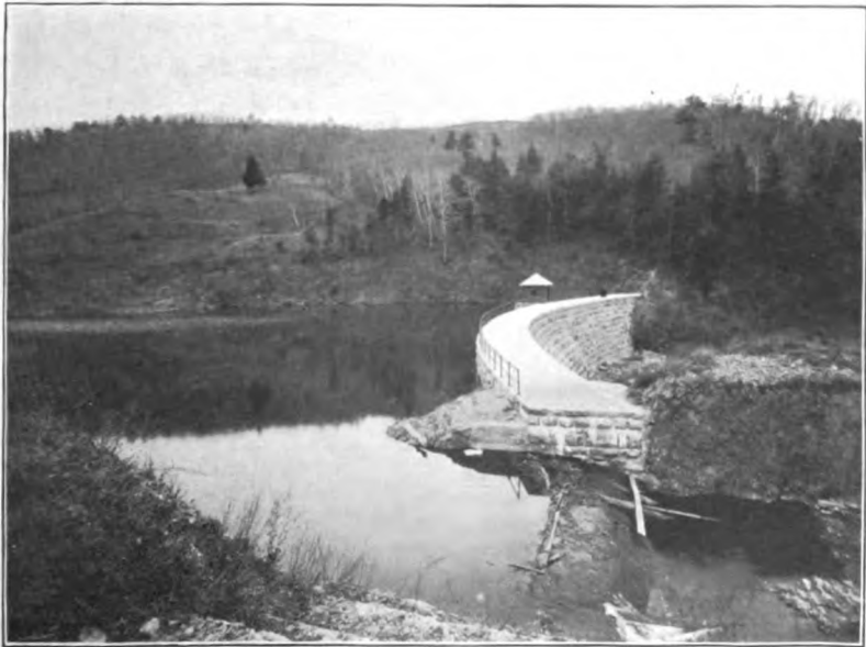
FIG. 2. Deepkill Dam and Reservoir, looking westerly.
