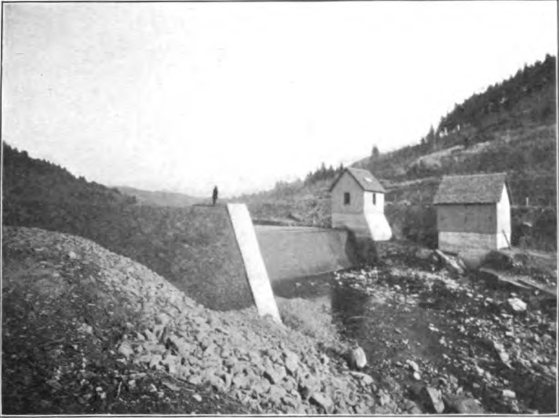
FIG. 1. Quackenkill Diverting Dam and Gate House.
