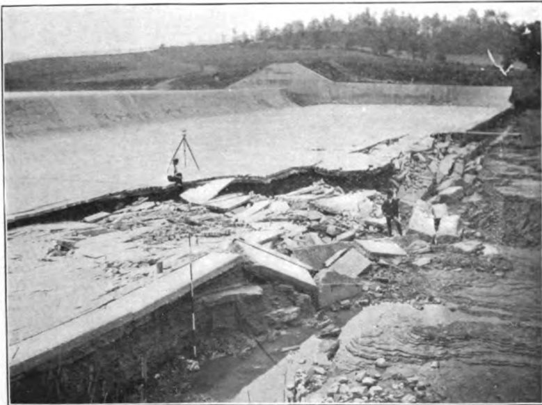
FIG. 2. Condition of Apron of Spillway Dam after the Flood of June 23, 1906.
