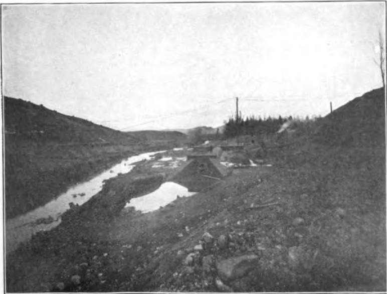
FIG. 2. Tomhannock Dam Site with Culvert Completed.
