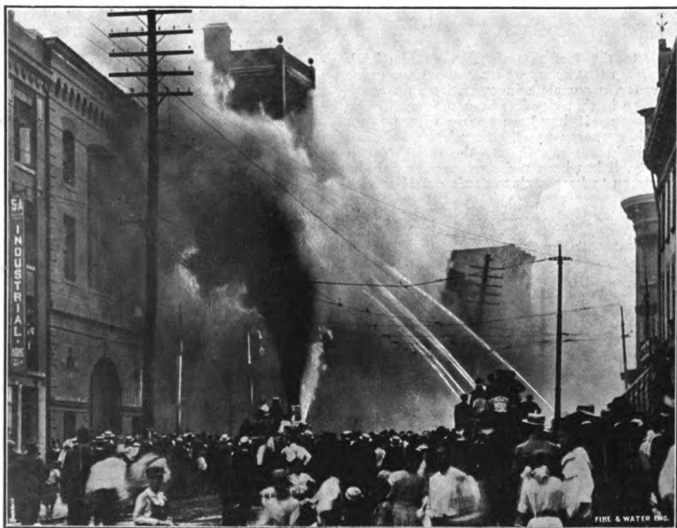
TROY, N. Y. FIRE DEPARTMENT IN ACTION AT COLLAR AND SHIRT FACTORY FIRE.
