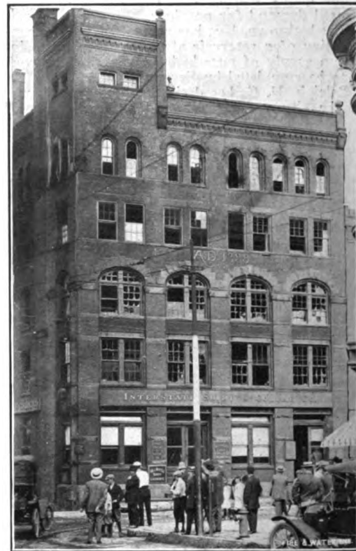
INTERNATIONAL COLLAR AND SHIRT FACTORY, TROY, N. Y., WHERE FIRE BROKE OUT.
