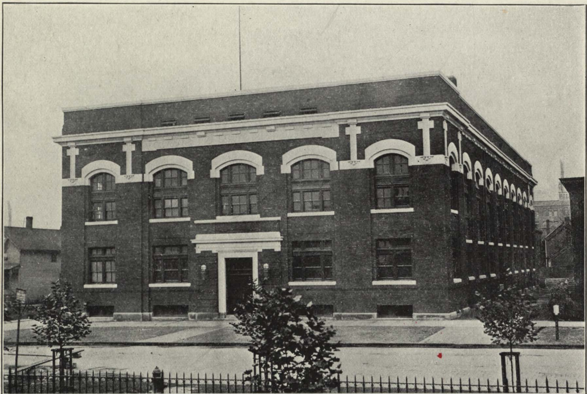
CLEVELAND HIGH PRESSURE STATION. (1108 Lakeside Avenue N. E.)
