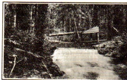
MEASURING WEIR ON BULL RUN
