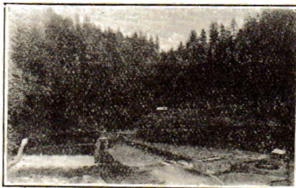
HEADWORKS ON BULL RUN
