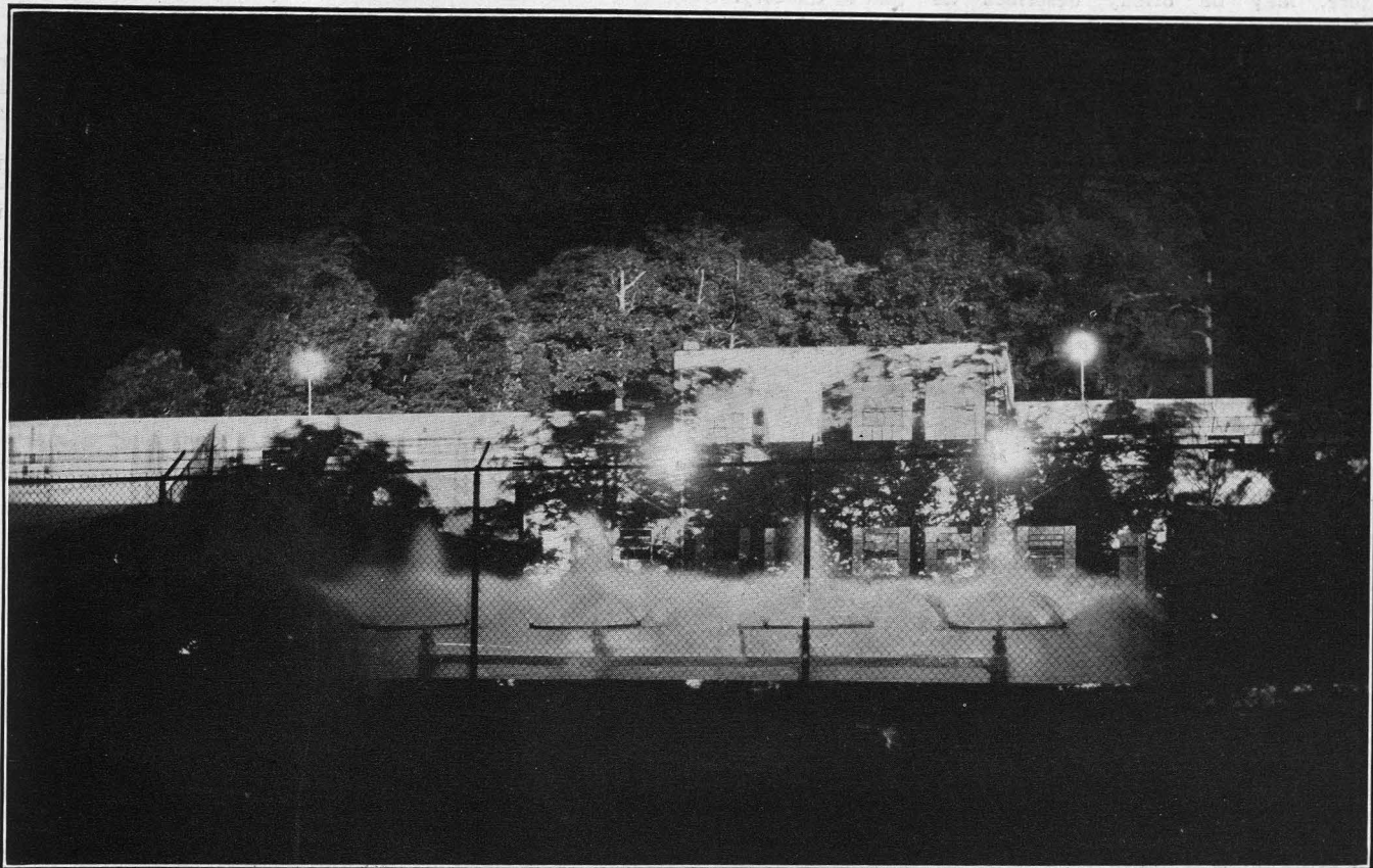
Night View of Plant Showing It Illuminated with Monticello Search Light. The Secondary Aerators are in the Foreground
