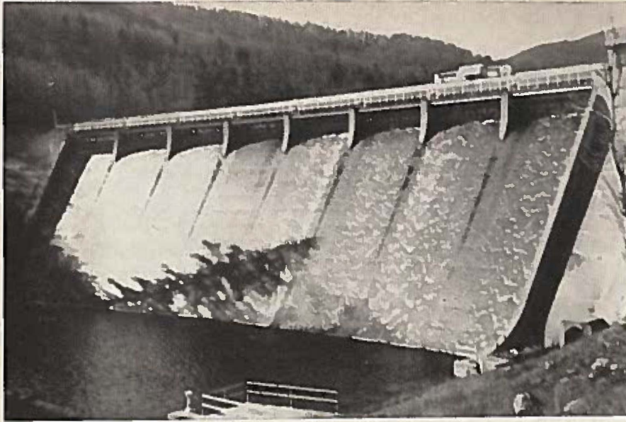
FIG. 3. UPSTREAM VIEW of Moorman's River Dam.
