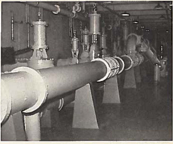
FIG. 6. SECTION of pipe gallery showing effluent controllers.
