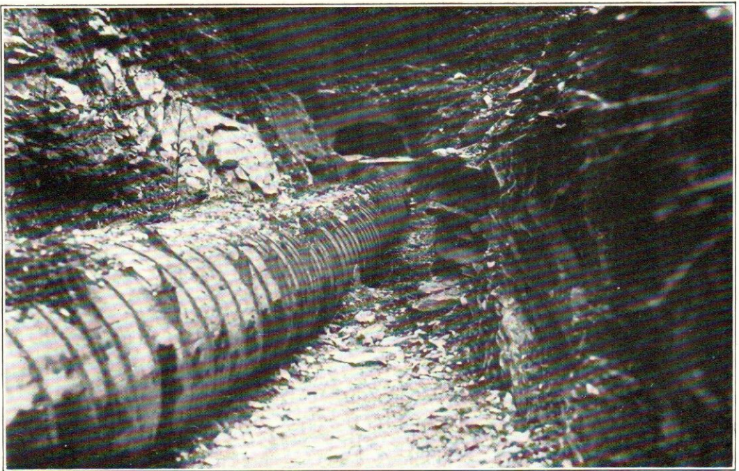
SECTION OF OLD WOOD STAVE CONDUIT
