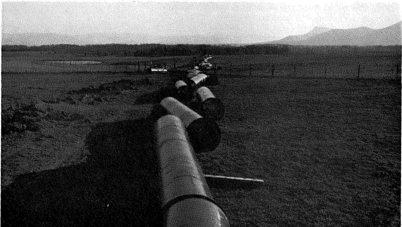
A cross-country stretch of LFC's 24-inch cast iron pipe awaiting installation between the filter plant and Middletown.
