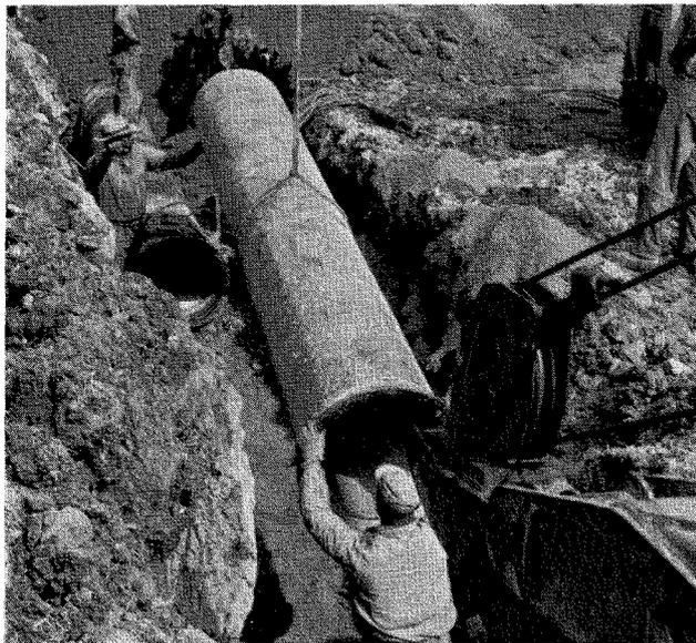
Construction workers lower a section of 24-inch pipe into the trench. Boyd and Goforth Construction Company are the contractors here.
