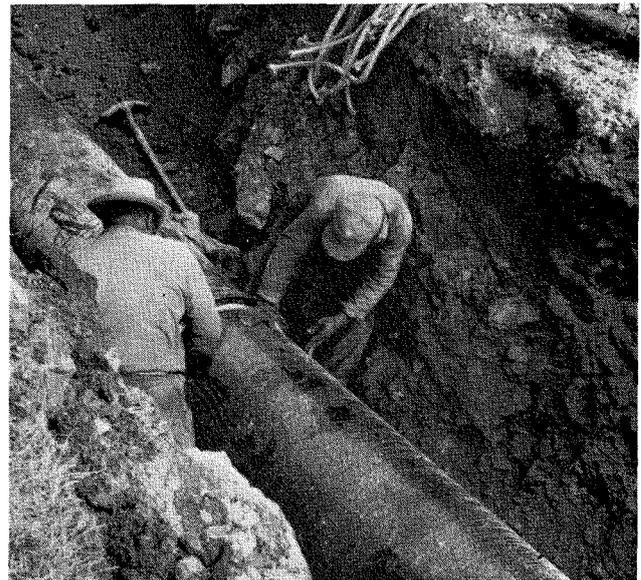
The operation being performed here is that of caulking a 24-inch bell and spigot joint prior to pouring a sulphur base compound.
