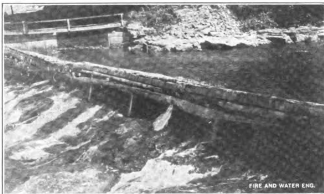
Fig. 1—Old Wood Crib Dam
