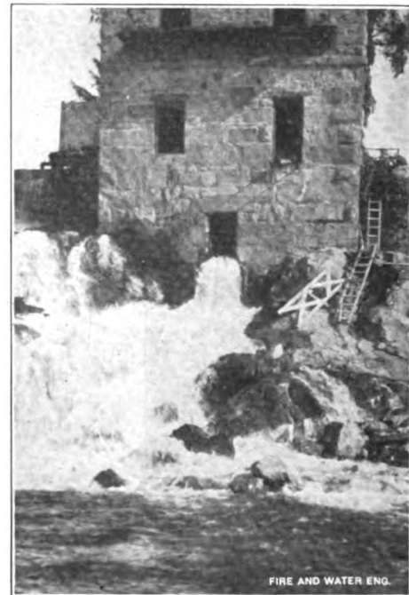
Fig 2—Rear View Old Pump House, Showing Discharge of Old Turbine
