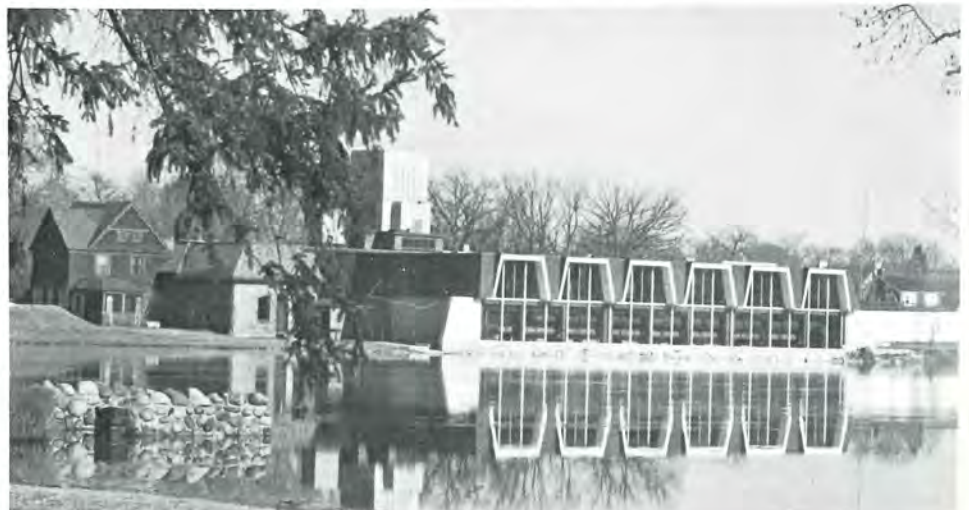
Water Treatment Plant on the banks of the Kankakee River (Ill.)
