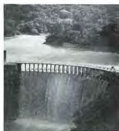
San Clemente Dam, owned and operated by the Monterey District of California American Water Company. Located in the mountains above the Monterey Peninsula it impounds water from the Carmel River.
