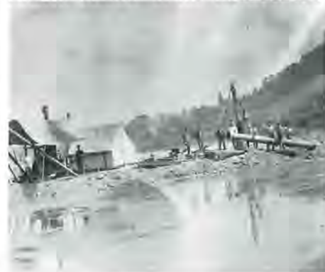
Installing a river crossing at Sayre, Pennsylvania, by means of a temporary earth fill.
