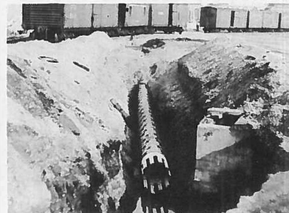
20" Untreated Continuous Stave Pipe
