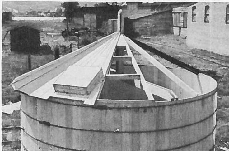
Conical Cover Showing Steps in Construction
