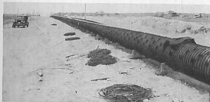
34" Creosoted Irrigation Pumping Line
