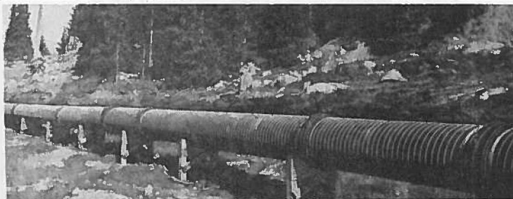
18" Pipe for Mine Tailings
