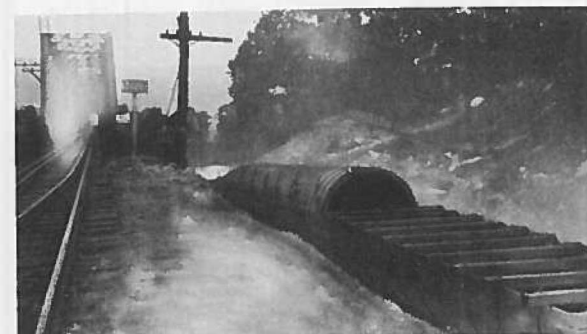
48" Flume to 48" Pipe, with Reducer to 42" Pipe
