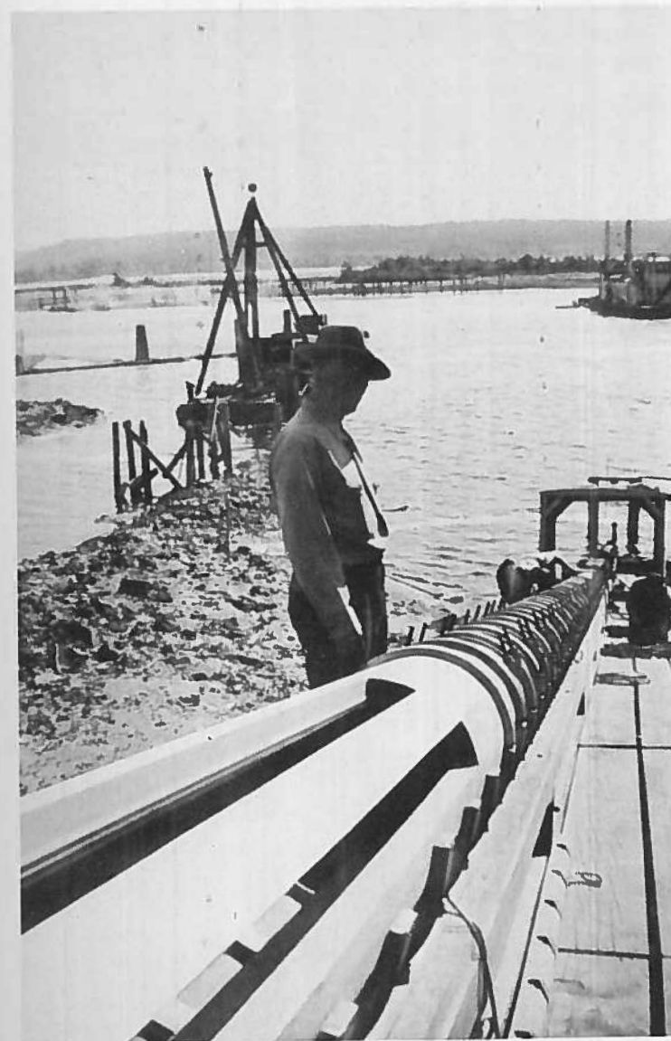
Ten Inch Continuous Stave Submarine Pipe Line shown on Launchway
