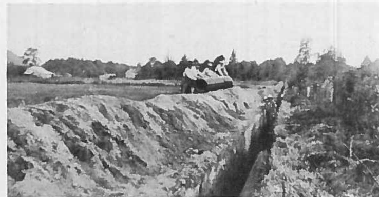
Installing 16" City Supply Line
