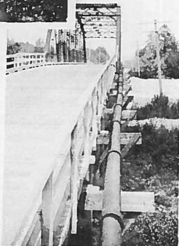
12" originally installed 1913, relaid 1933; picture taken 1941.
