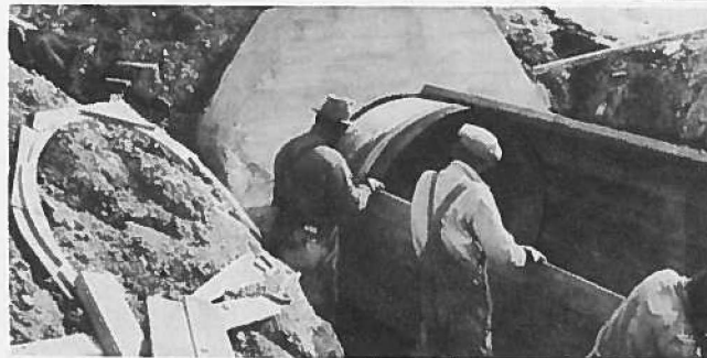
60" Wood to Steel Connection
