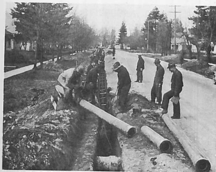
Laying FEDERAL Wire-Wound Pipe Distribution System
