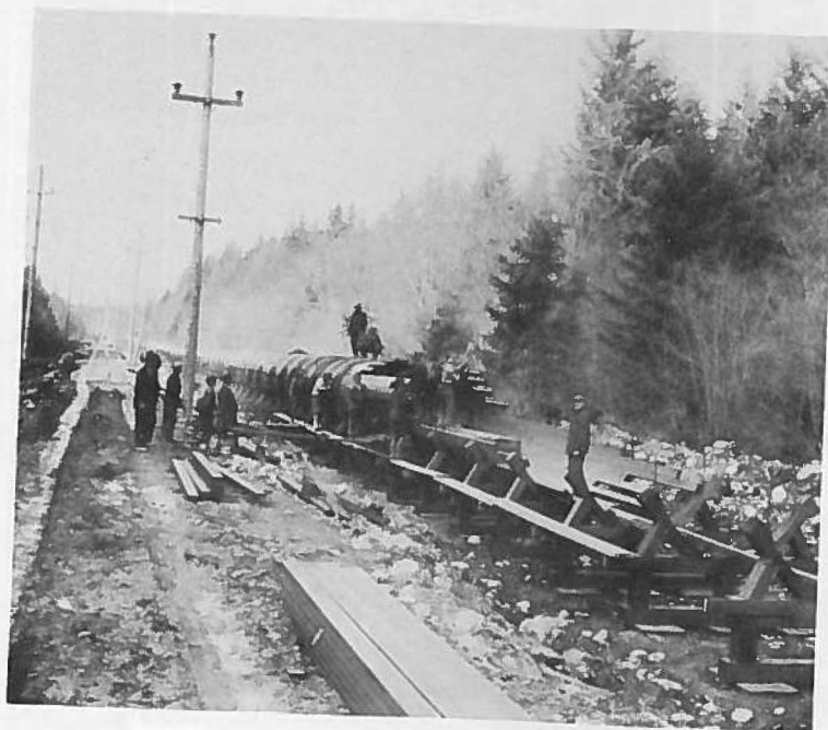
FEDERAL 6½-foot diameter Creosoted Fir City Supply Line
