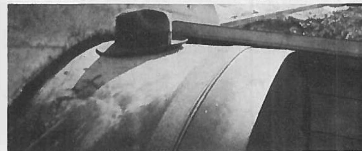
Close-up of Wood to Steel Connection, Showing Rope Gasket
