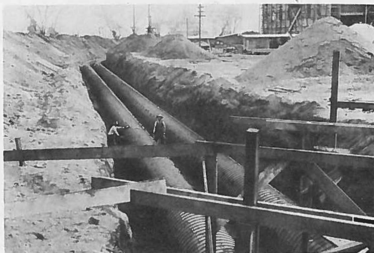
Parallel Lines of 48" Pipe
