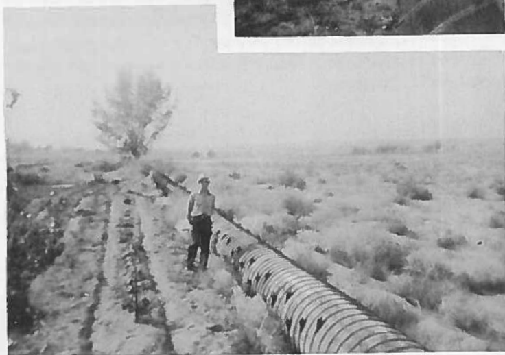
Same 50" Creosoted Pipe dismantled and reconstructed in 1939—100% sound.
