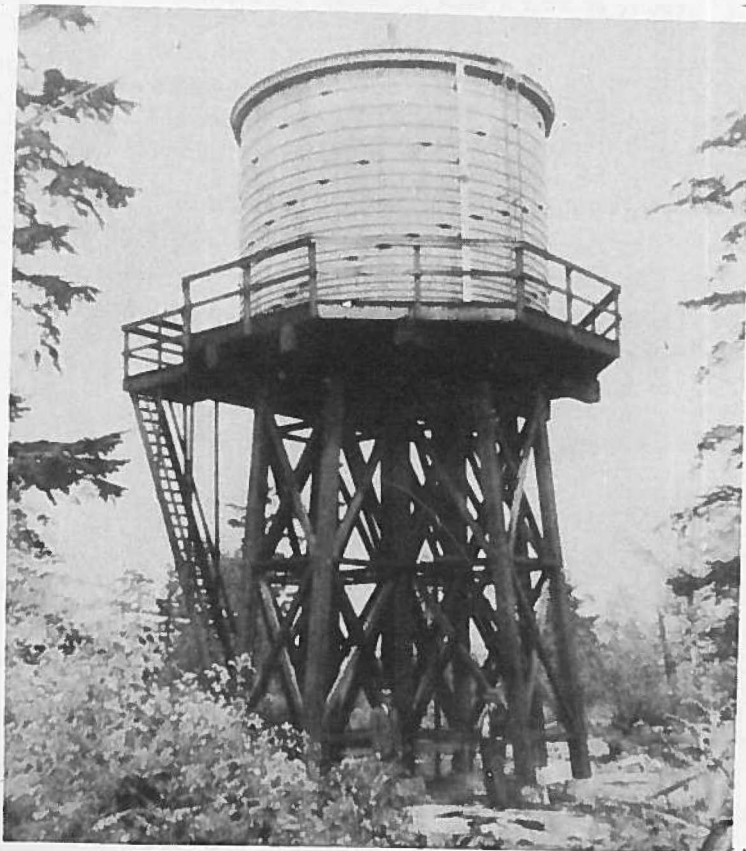
34,000-gallon Cedar Tank on 24-ft. creosoted Fir Tower
