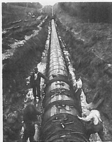
Banding crew working on 54" Creosoted Pulp Mill and City Supply Line. Opening in distance was "buckled in" later.
