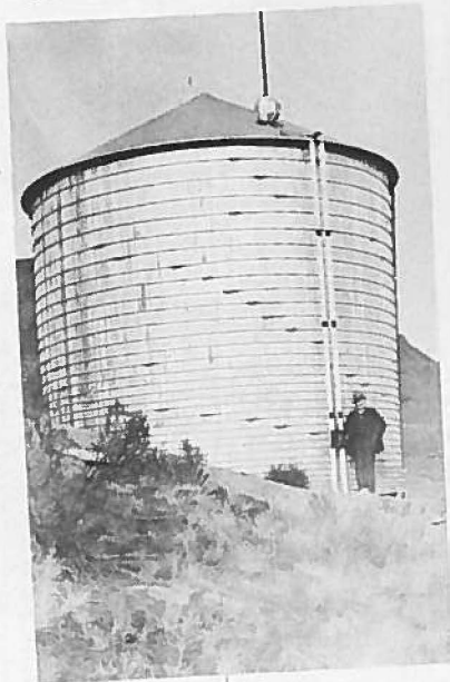
33' x 20' Headed Tanks with 10" and 14" FEDERAL Wire-Wound Pipe.
