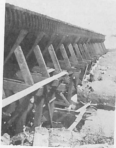
Side view of 16-foot Flume, showing creosoted cradles and sub-structure.
