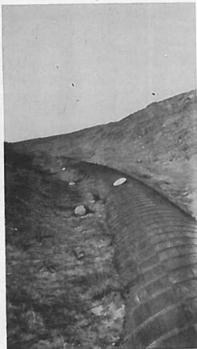
Same 50" Creosoted Pipe dismantled and reconstructed in 1939—100% sound.
