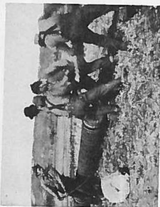
Installing 6" FEDERAL Untreated City Supply Line along Highway.
