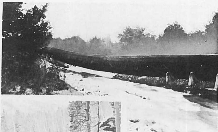
TOP: 78" undermined for 100-foot span, but carried full load for some time.
