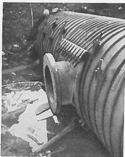
Flanged Saddle for Blow-off on 34" Continuous Stave Pipe
