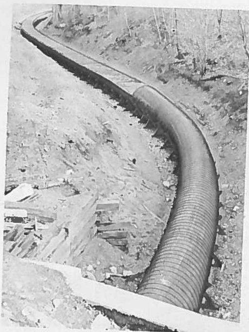
Curved Pipe and Flume
