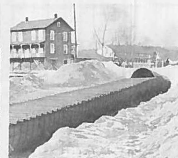
84" Flume to 84" Pipe, and reducing to 66" Pipe
