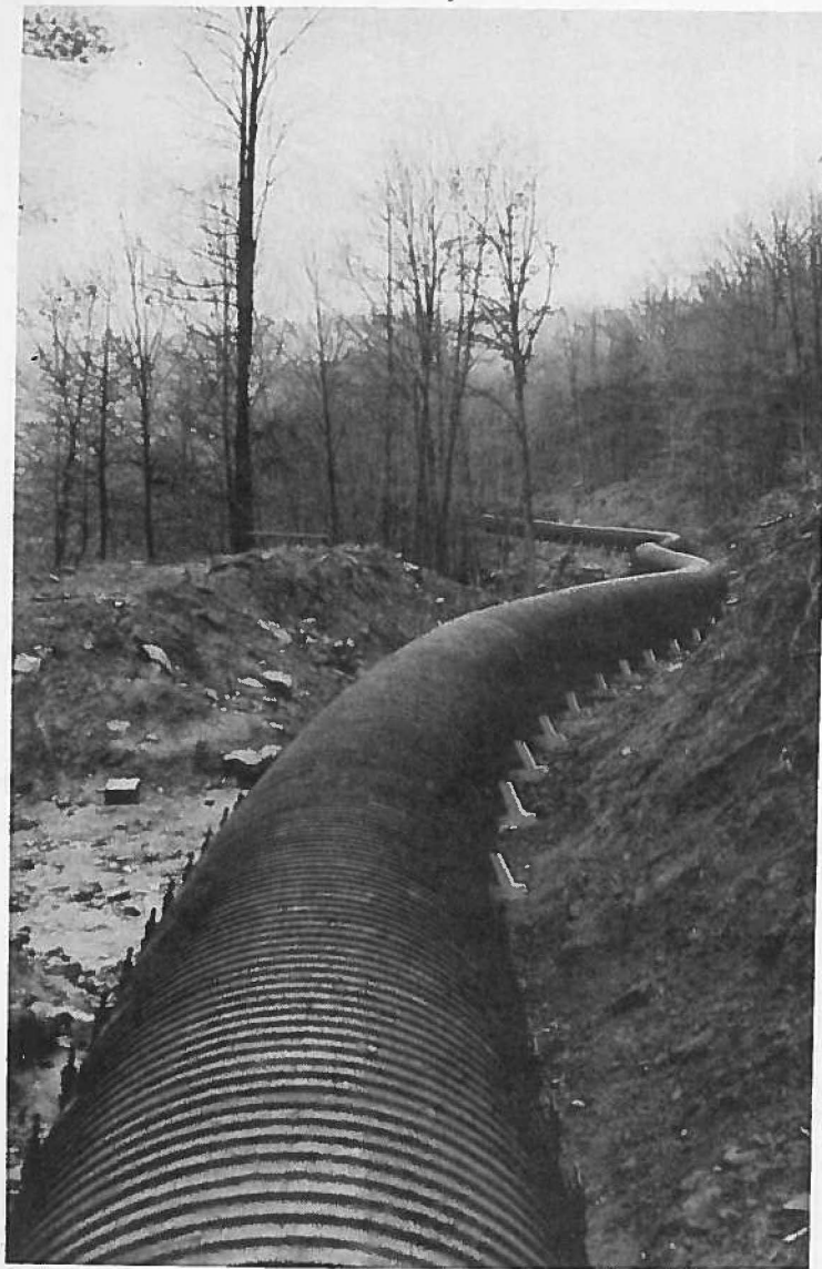
84" Pipe for Water Power Plant
