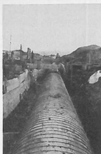
60" Creosoted Wood Outfall Sewer installed above ground in 1918.
