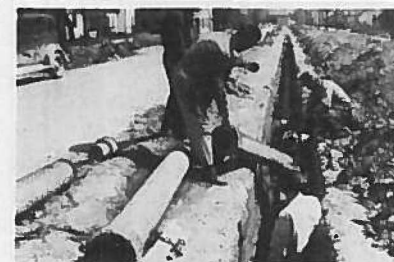
Laying Wire-Wound Pipe
