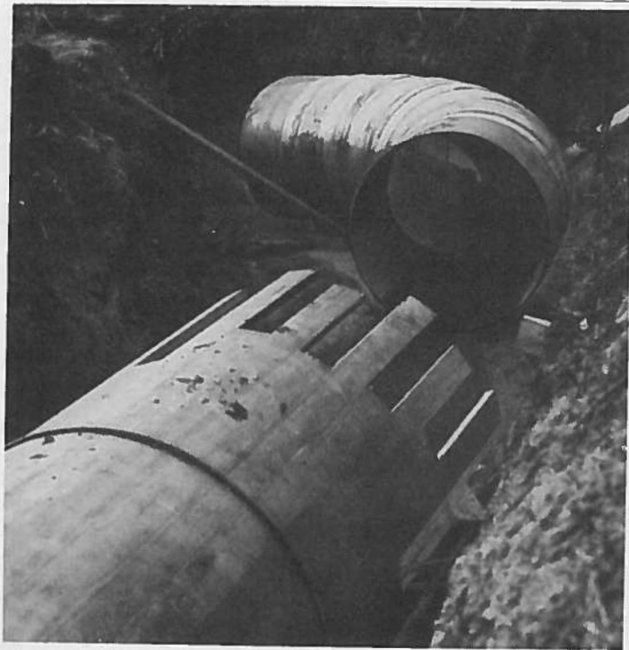
Welded Steel Bend, Ready for Connection
