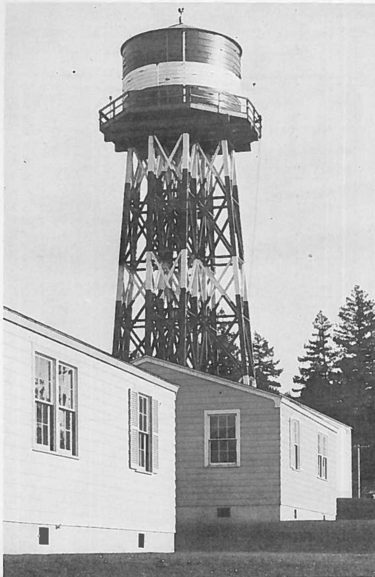
50,000 gallon Douglas Fir Tank on 75-foot Timber Tower
