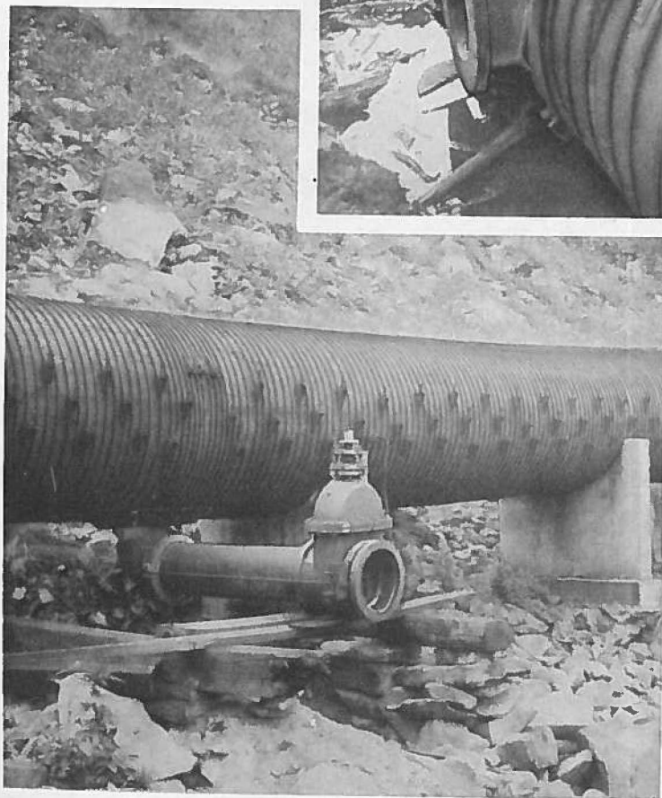
Hub End Blow-off with tie rods on 38" Pipe
