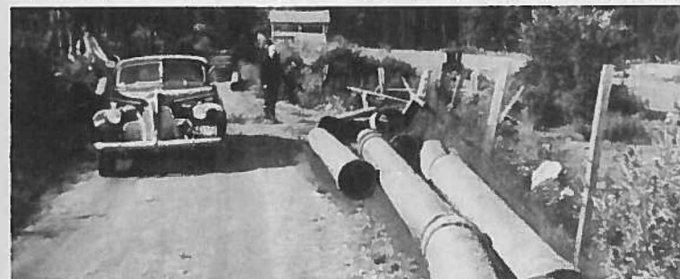
Preparing to install 18" Wire-Wound Pipe
