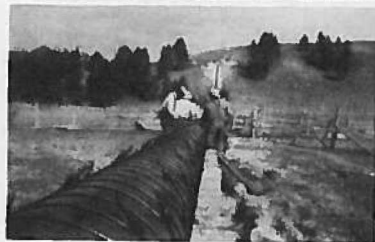
Building 22" Creosoted Irrigation Siphon
