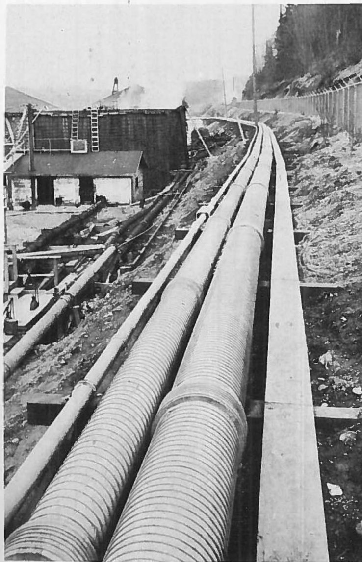
Wire-Wound Pipe Installed in Cradles shown on previous page
