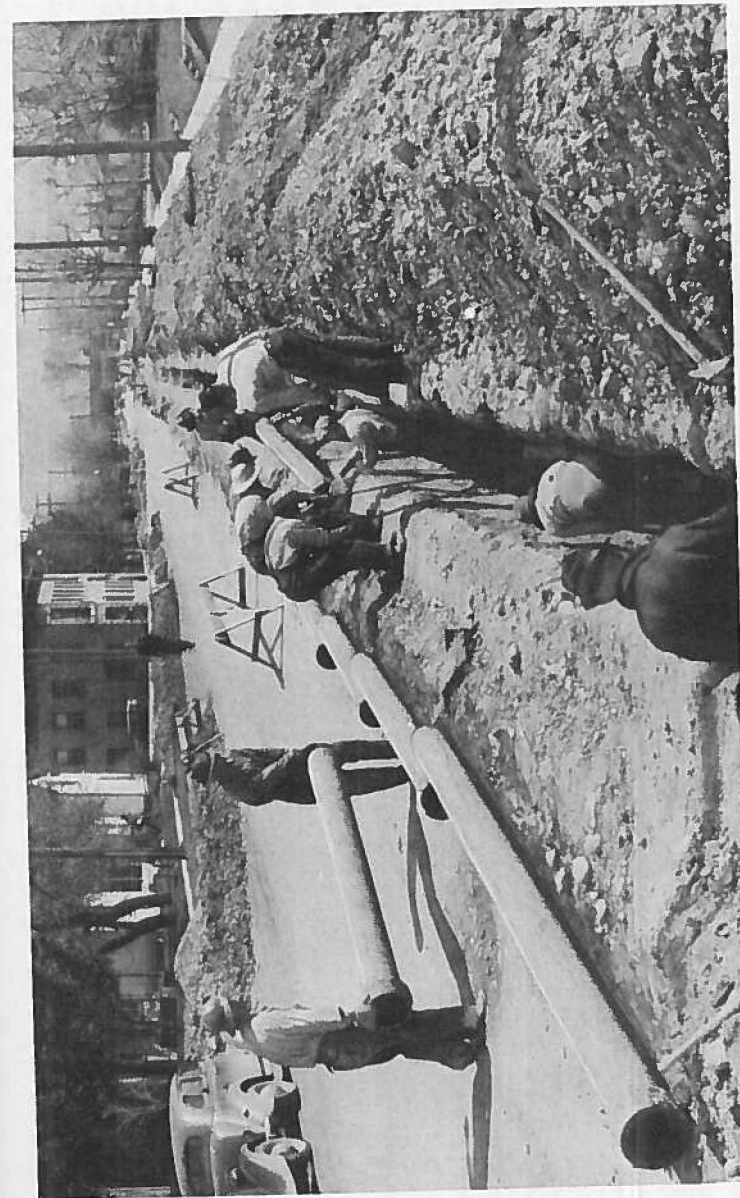
Laying 6" Wire-Wound Pipe
