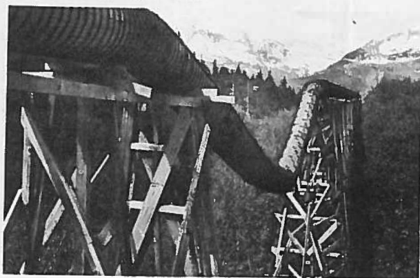
BELOW: Trestle failure under 95 feet of 36" pipe, resulting in 25-foot sag. Service continued one month at 30 pounds internal water pressure.
