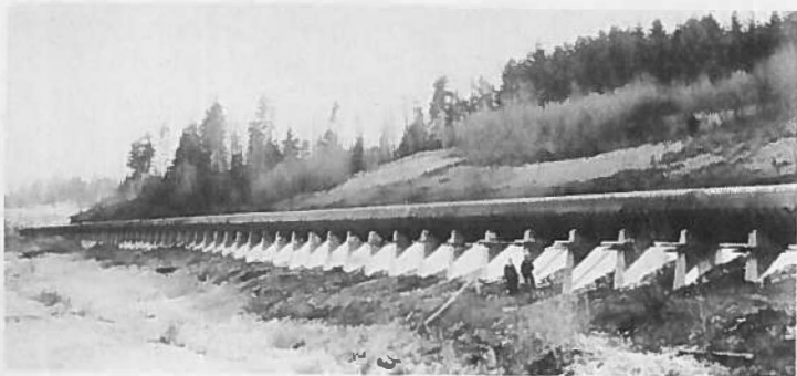
Reinforced Concrete Cradles
