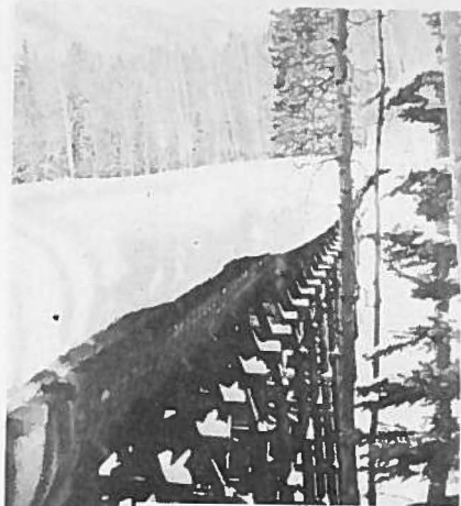
BELOW: Trestle failure under 95 feet of 36" pipe, resulting in 25-foot sag. Service continued one month at 30 pounds internal water pressure.
