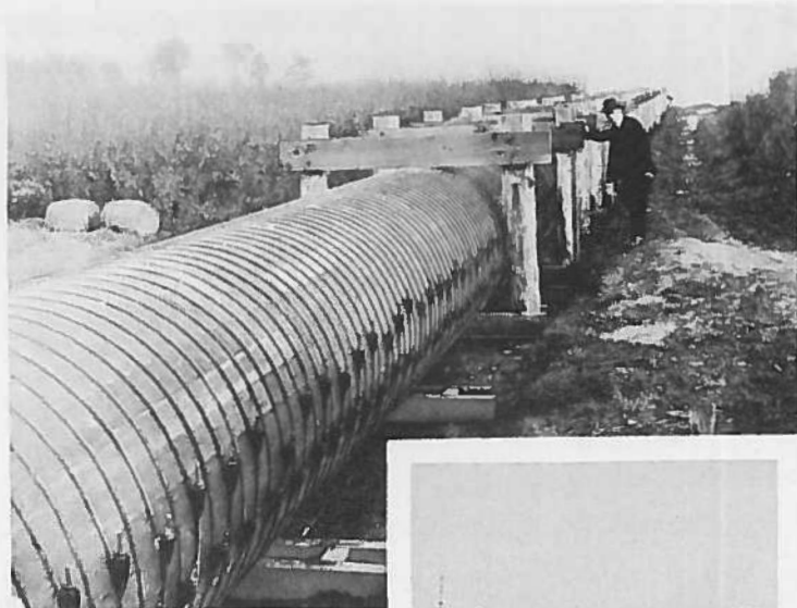
60" Creosoted Wood Outfall Sewer installed above ground in 1918.
