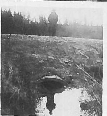
60 Feet of 48" Culvert, assembled on bank and rolled into stream
