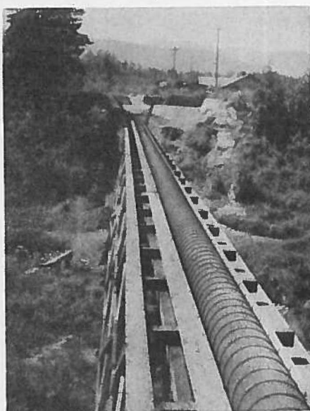
36" Creosoted Sewer Pipe at large sewage disposal plant.
