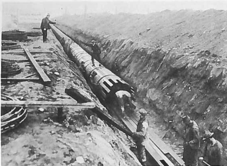
Typical View of Continuous Stave Pipe Erection, showing a 52" creosoted City Supply Line.
