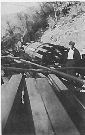
Starting construction of a 48" Wood Pipe for Water Power—pipe to be built in each direction.
