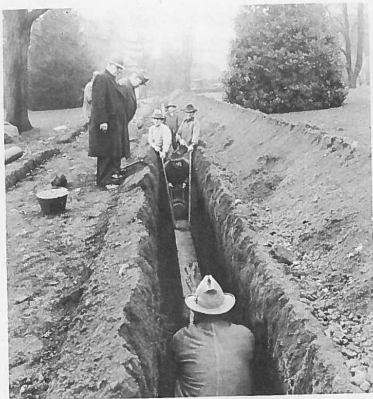
Laying FEDERAL Wire-Wound Wood Pipe in residential district
