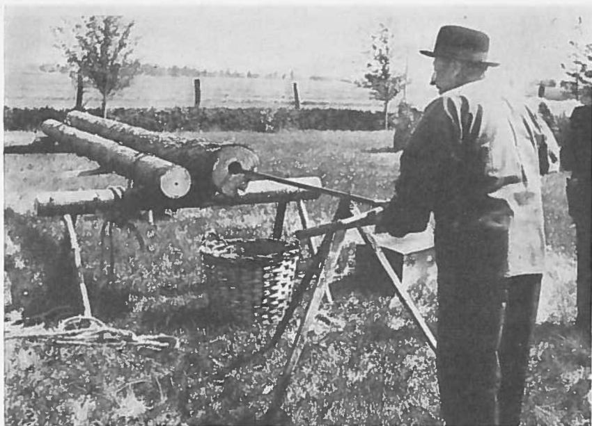
Fig. 2. Boring of pine trunk pipes for water mains in Sweden, Province of Västergötland, in 1945. The same method of manufacture was used as early as at the beginning of the 19th century, when wood pipes of this type were common in this part of the country. (This photograph has been published in the Västra Sveriges Lantmannatidning ).
