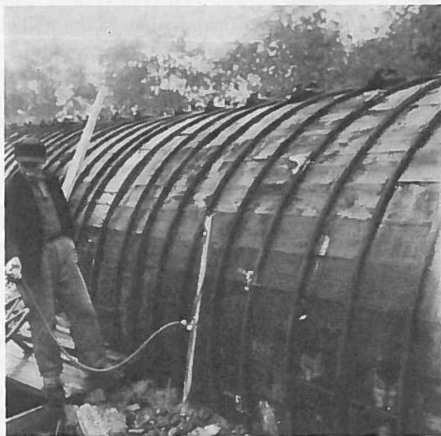
Fig. 11. View of test set-up for strain measurements made on the wood-stave pipe at the Sikfors Hydro-Electric Station. The tensometers were attached to the bands at several points on the circumference of the pipe. The water pressure was measured by means of a mercury manometer which communicated with the water in the pipe through a rubber hose. At low pressures, the water level in the pipe was indicated by a glass tube gauge.
