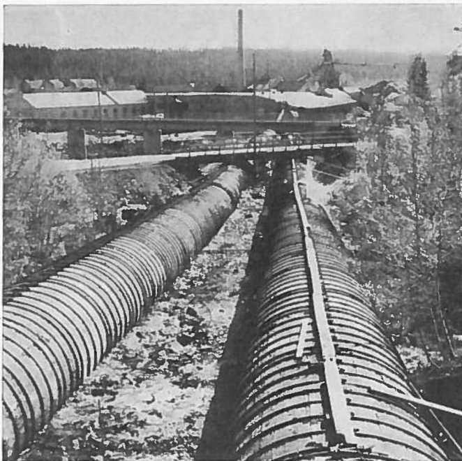
Fig. 16. Two wood-stave pipes at the Äggfors Hydro-Electric Station after 35 years of operation. On account of the presence of shrubbery in the neighbourhood of the pipe and because of careless maintenance, the pipe has been damaged by decay, particularly in the longitudinal joints between the staves (cf. the two pipes at Sikfors which are equally old, see Fig. 5).
