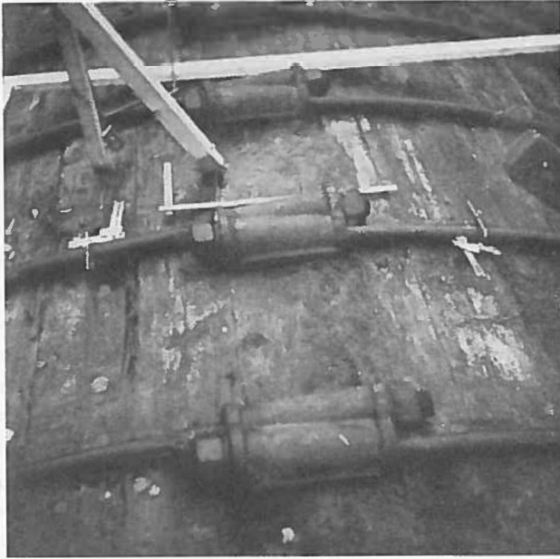
Fig. 12. Strain measurements on the wood-stave pipe at the Äggfors Hydro-Electric Station. Tensometers attached on the upper side of the pipe.
