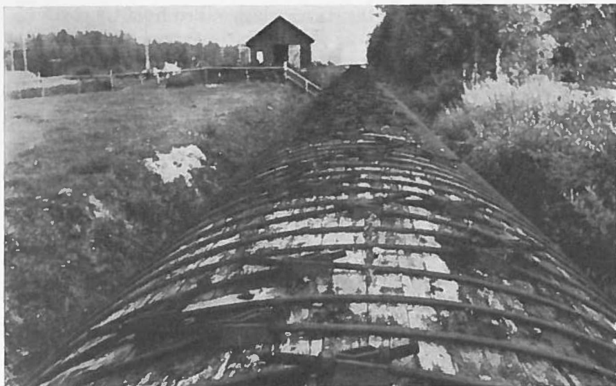
Fig. 15. Embedded section of the wood-stave pipe at the Gideåbruk Hydro-Electric Station, 3.2 m in diameter. This pipe has been in operation more than 30 years. The upper surface of the pipe is slightly damaged by decay. The shoes are of the eccentric type.
