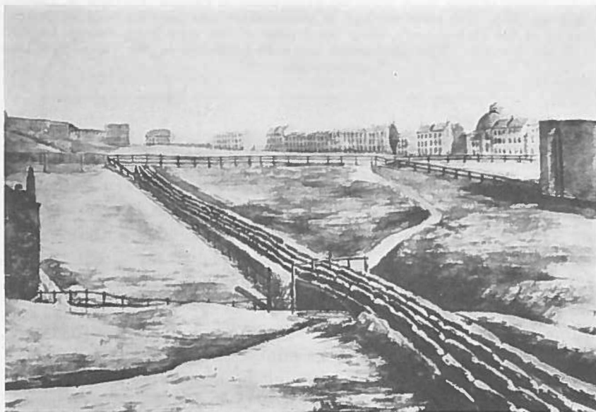
Fig. 1. An old water main in London. The construction of these mains was begun in the 17th century. The pipes were made of bored tree trunks. Several pipes were connected in parallel in order to increase the carrying capacity of the main. (Reproduced from a publication of the Metropolitan Water Board entitled «The Water Supply of London» (67).)
