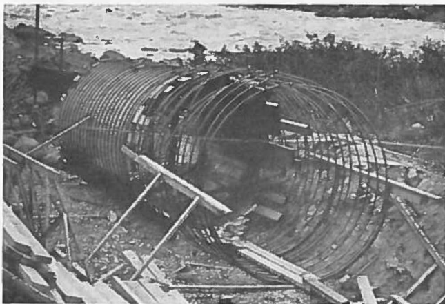
Fig. 13. One of the two wood-stave pipes at the Sikfors Hydro-Electric Station in process of construction in 1913. The diameter of the pipe is 3.2 m. Cf. Fig. 5.
