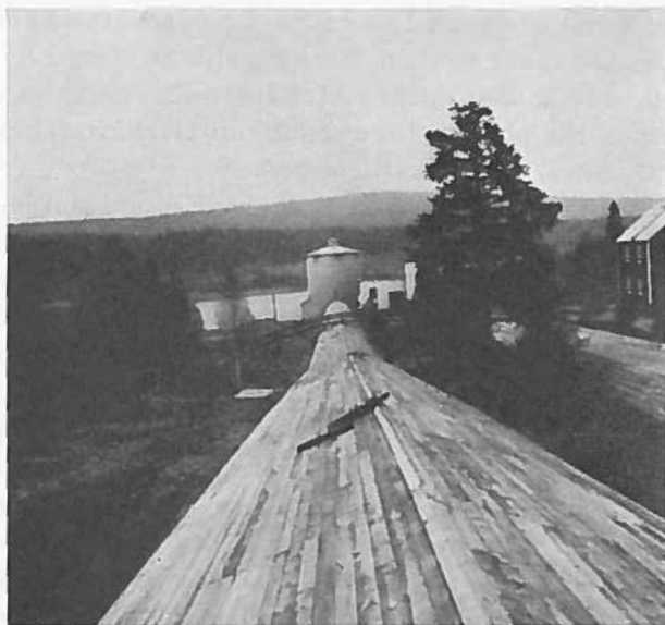
Fig. 14. The large wood-stave pipe at the Harrselsfors Hydro-Electric Station, 3.0 m in diameter. In view of the operating experience with the two older, smaller pipes (visible on the right), this pipe has been completely enclosed by plank walls in order to protect it from freezing.
